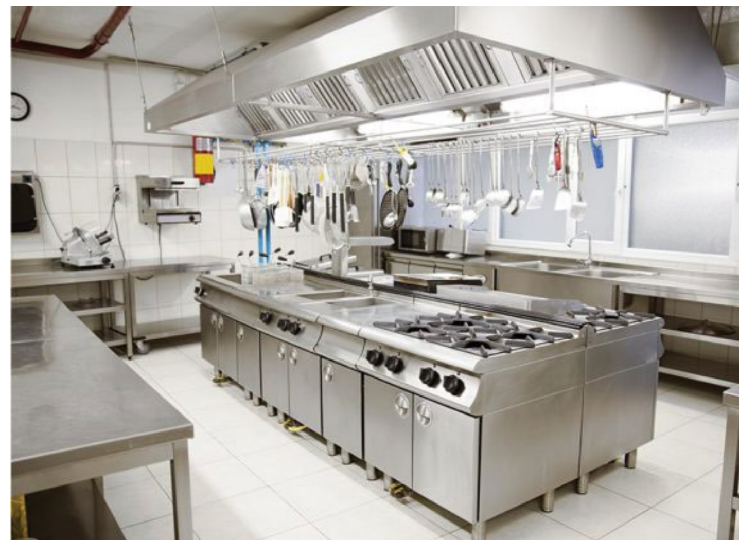
Stainless steel is the ultimate material for the hotel or restaurant kitchen on account of its hygienic qualities.
